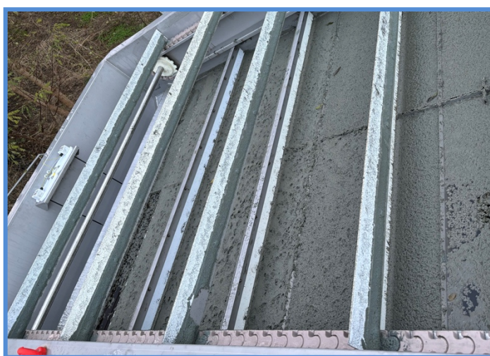
Photo 2: DAF Sludge (8-10% DM) and skimmer
