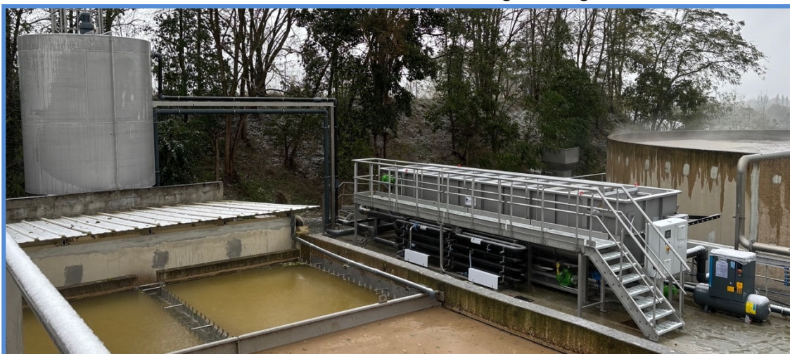
Photo 1: Dissolved Air Flotation DAF with Flocculator and sludge holding tank
